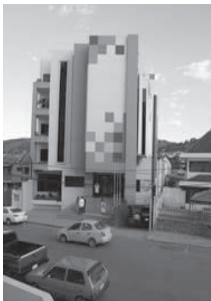
Hospital Monte Sinaí, Torre I
