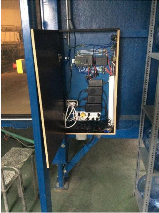
*Figura A.18 PLC instalado*
