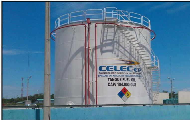
Figura 22 Tanque de Fuel-Oil
