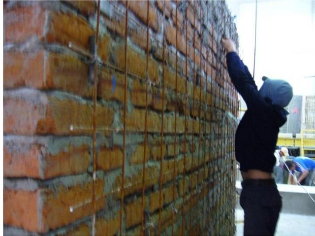
Fig. 4.2 Malla electro soldada ARMEX-R188.
